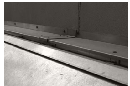
TRXM ● ● ● Flat Curb 6-24" [150-600mm] ±50% to ±100% / Seismic
